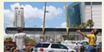
Preparing to fly the beam that was signed by more than 500 community members at the December 2007 groundbreaking
